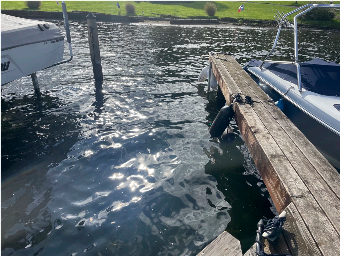
Photo 6 - Existing slip looking landward.
